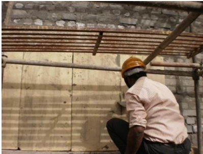
Rigid External Thermal Insulation Composite System
