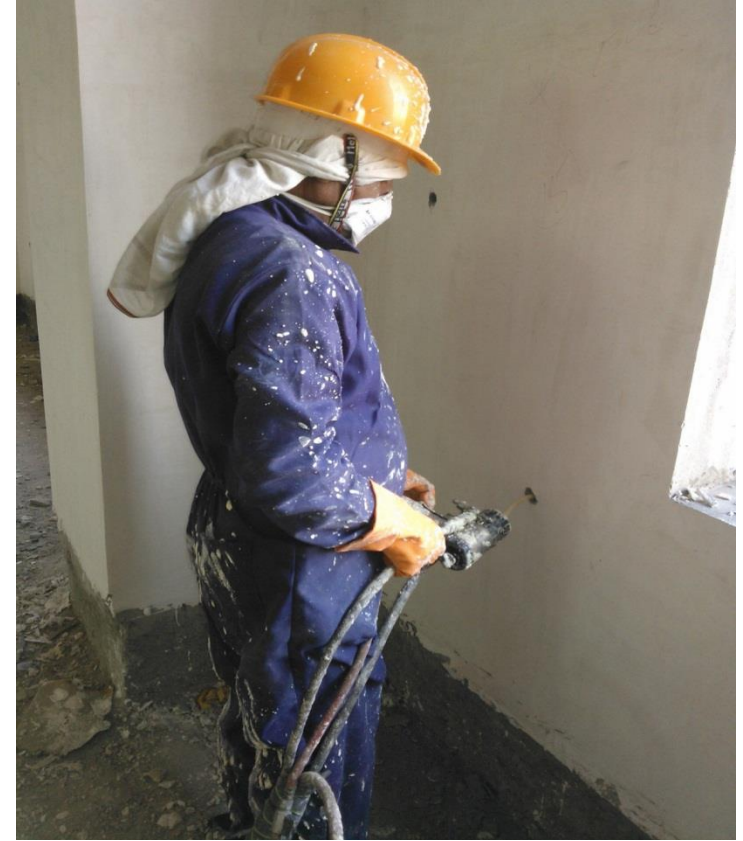
CAVITY WALL INSULATION WITH PUF CAST-IN-SITU
