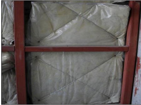
External Wall Insulation with Fibrous / Rockwool slabs
