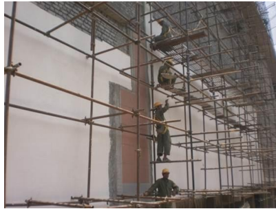
Rigid External Thermal Insulation Composite System
