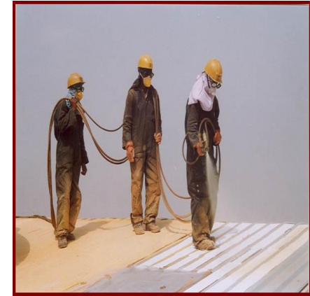
Rigid / PU External Roof & Wall Spray Insulation
