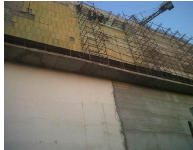
Rigid External Thermal Insulation Composite System
