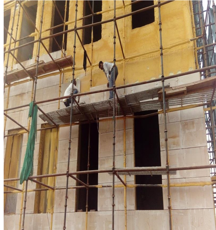
PUF SPRAY INSULATION WITH STONE CLADDING
