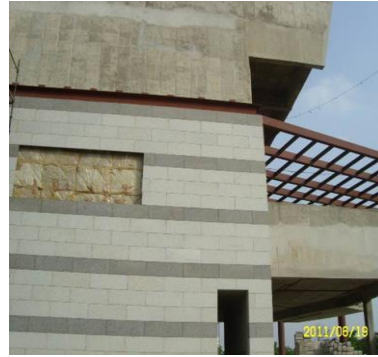
External Wall Insulation with Fibrous / Rockwool slabs
