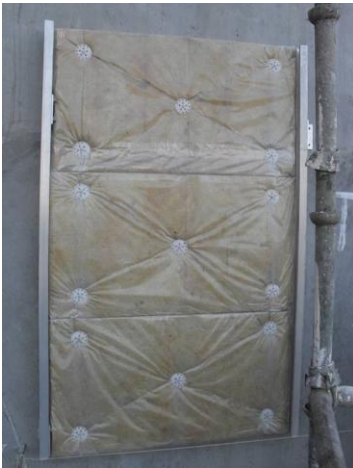
External Wall Insulation with Fibrous / Rockwool slabs
