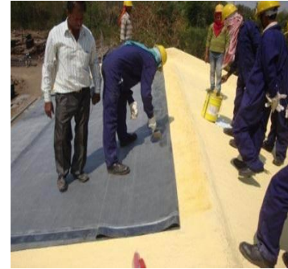
Rigid Roof Insulation with water proofing membrane
