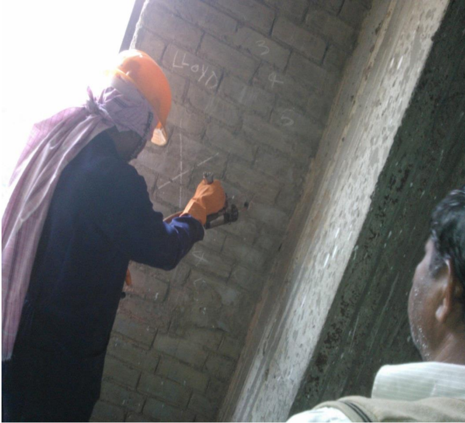
CAVITY WALL INSULATION WITH PUF CAST-IN-SITU
