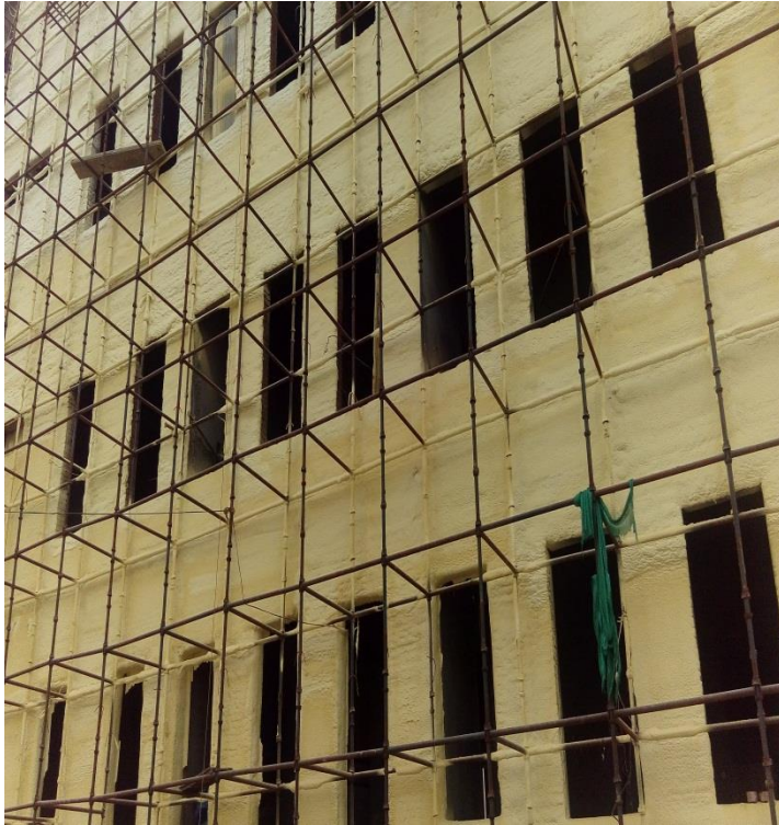
PUF SPRAY INSULATION WITH STONE CLADDING
