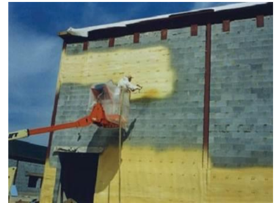
Rigid / PU External Roof & Wall Spray Insulation
