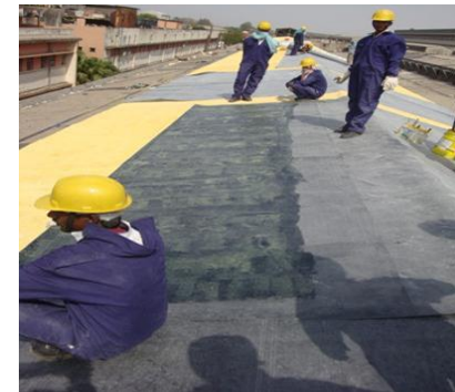
Rigid Roof Insulation with water proofing membrane
