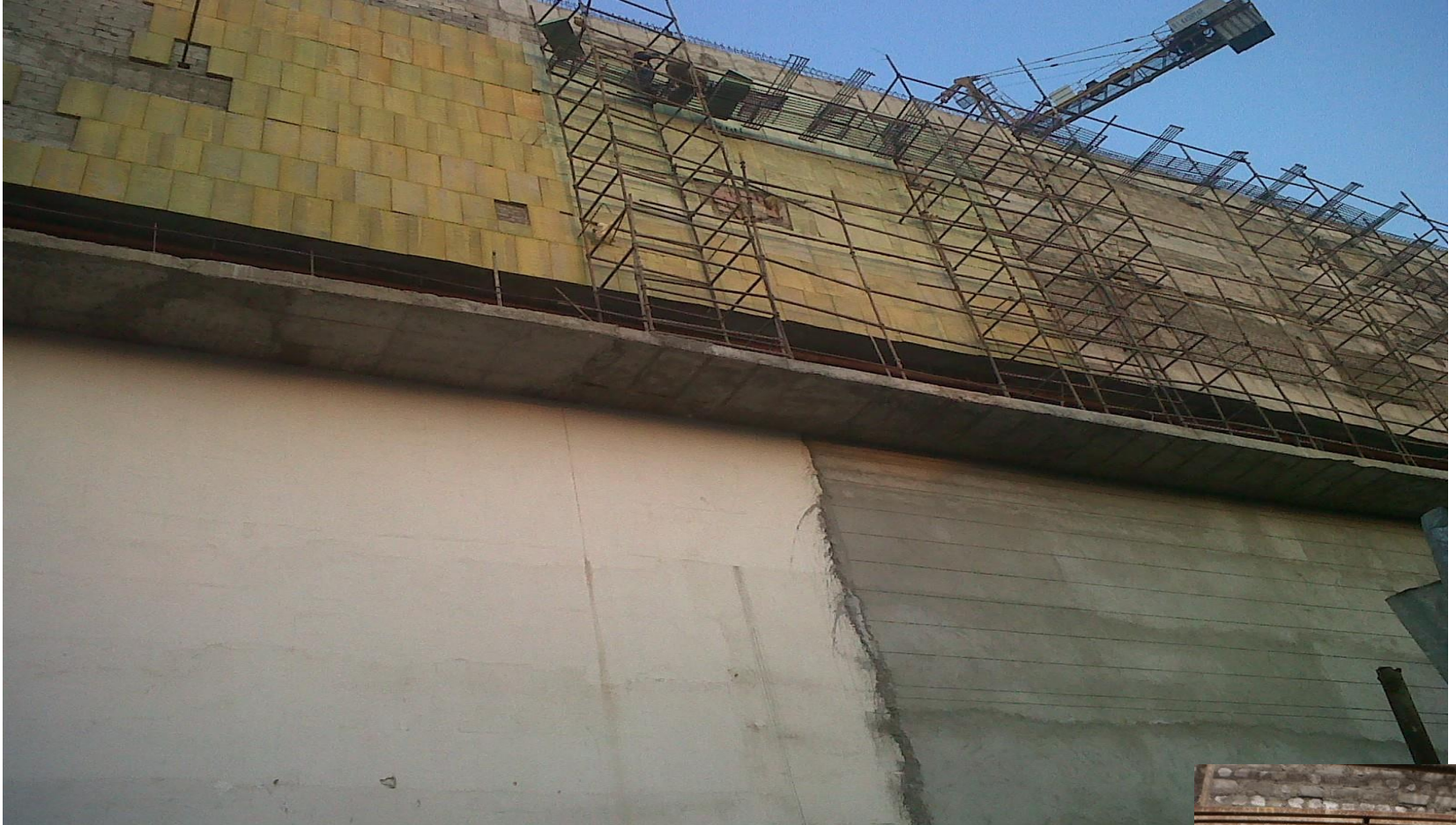
WALL INSULATION WITH PUF / PIR SLABS
