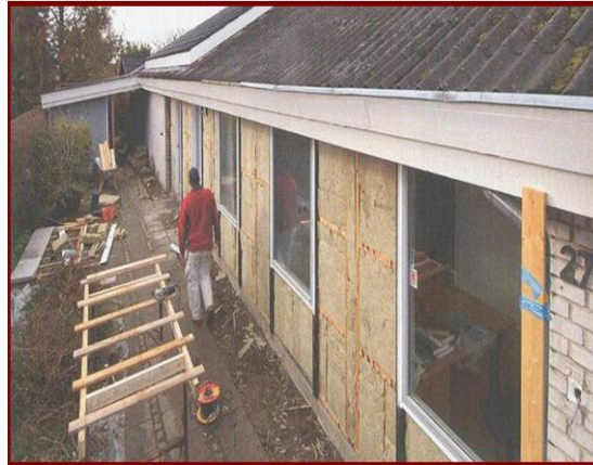
External Wall Insulation with Fibrous / Rockwool slabs
