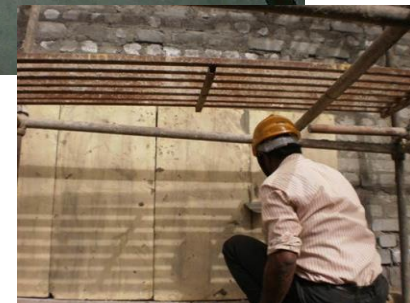
WALL INSULATION WITH PUF / PIR SLABS
